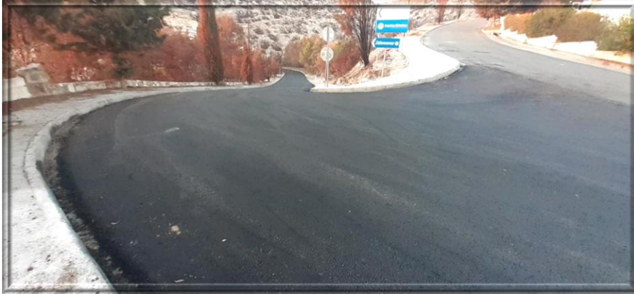
(Other roads have also had new tarmac laid)
